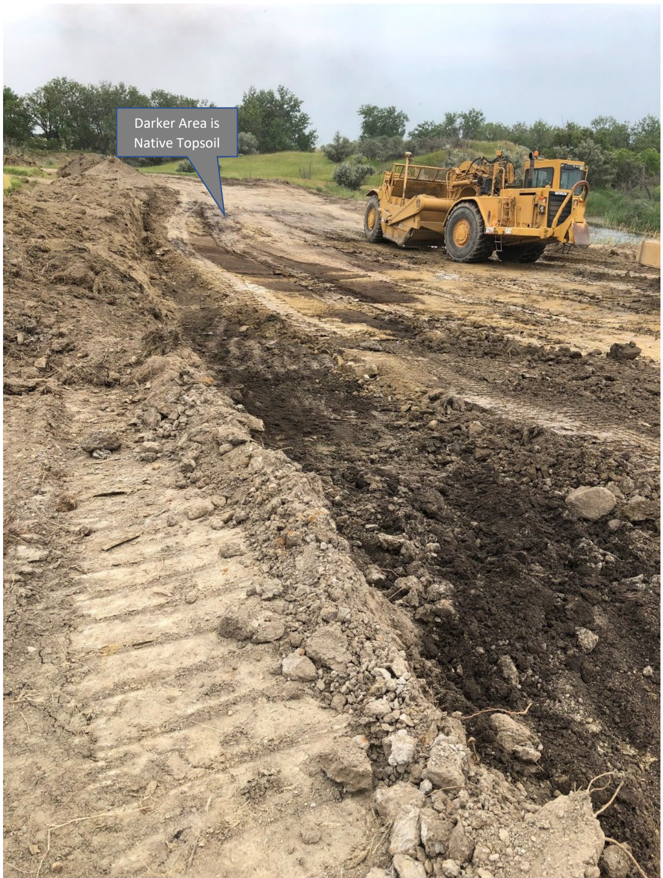
Figure 11: Original topsoil was exposed and salvaged along the north highwall in the West Youngtown Tract.
