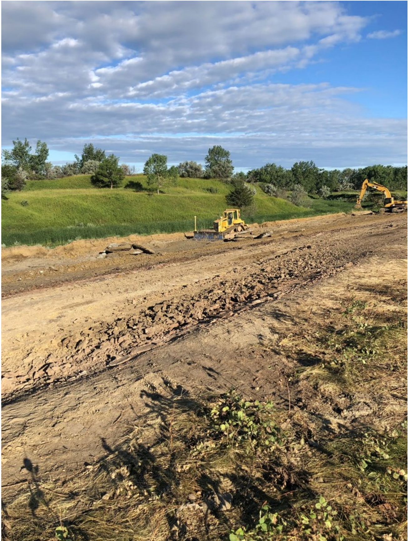
Figure 16: Dozing the excavated rock ledge in the East Youngtown Tract.
