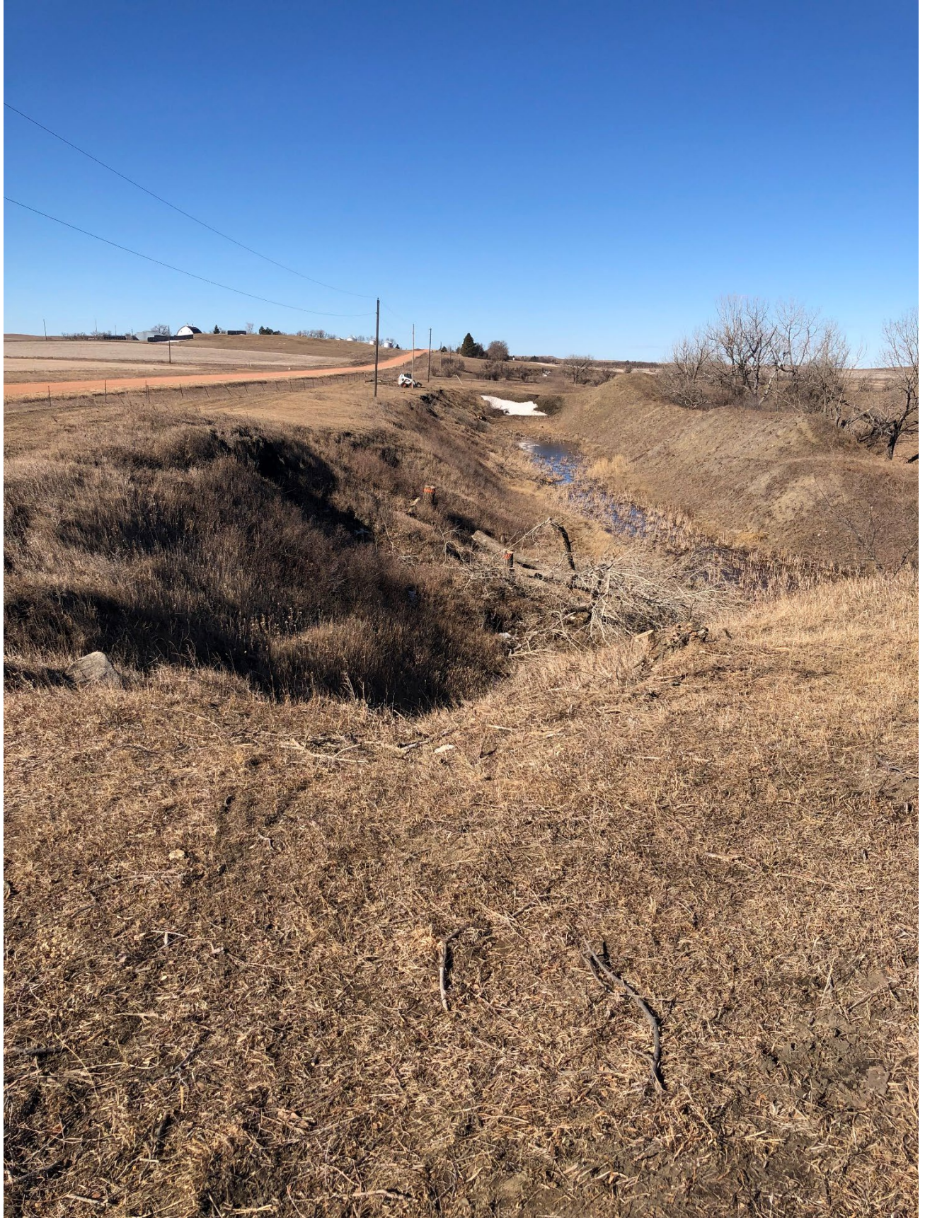
Figure 3: Trees felled along the East Youngtown highwall.
