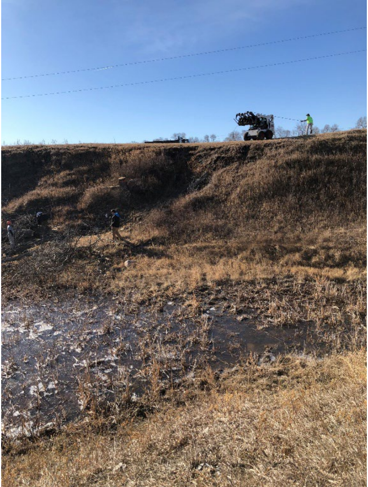
Figure 4: Tree removal operations in the East Youngtown's pit.
