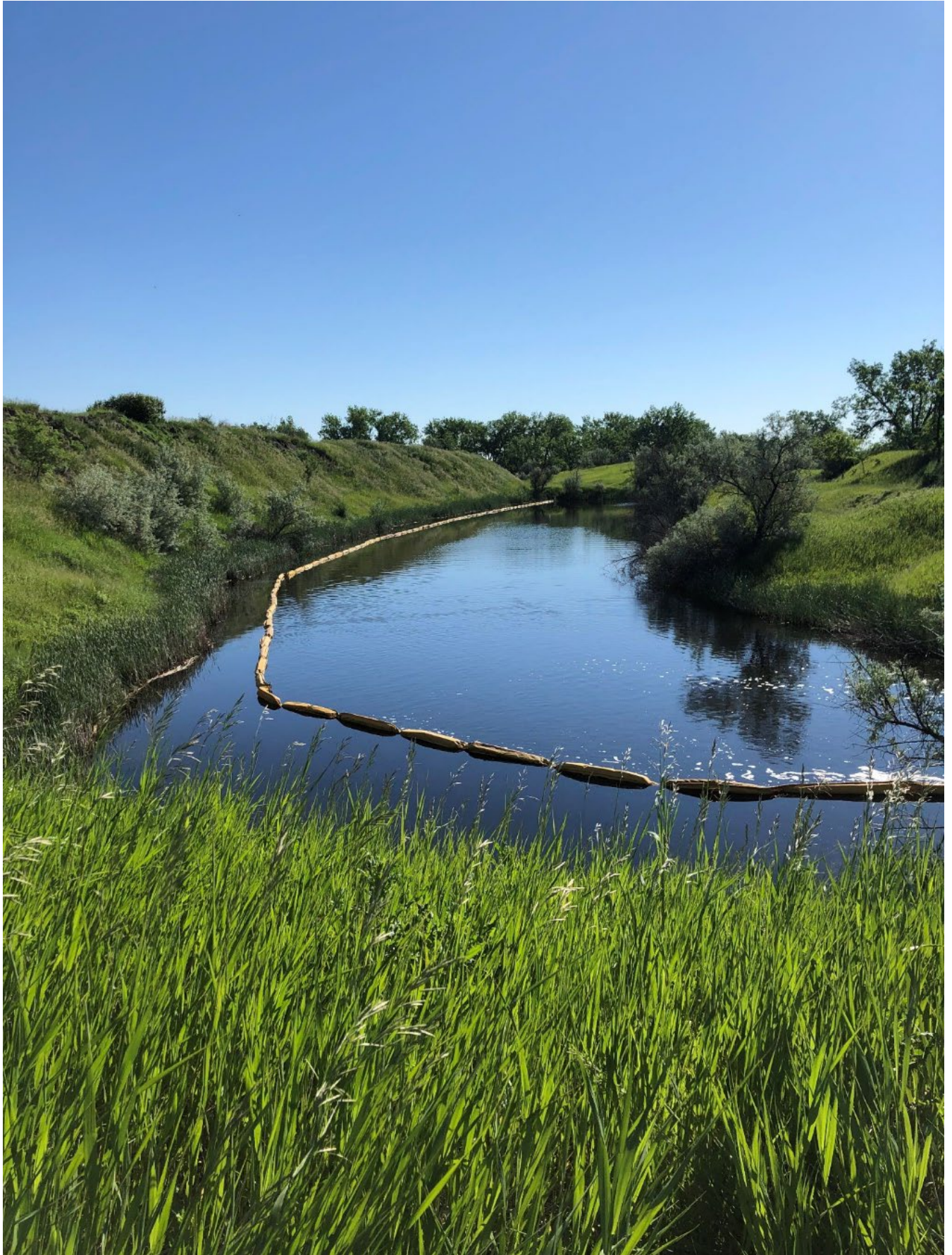
Figure 6: A turbidity curtain was installed in the pit pond along the north highwall.
