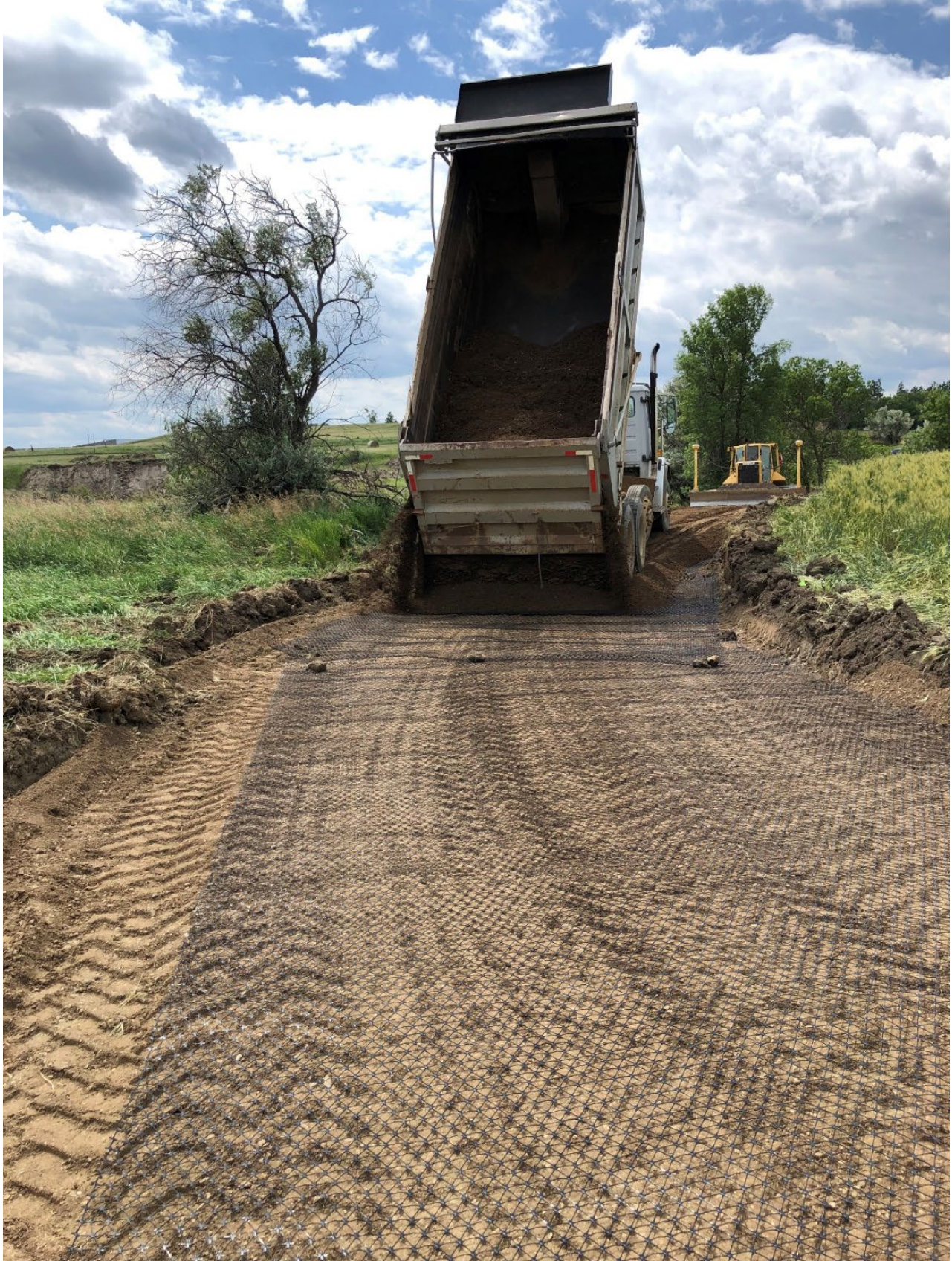
Figure 9: Constructing the temporary haul road/topsoil bridge in the West Youngtown Tract.
