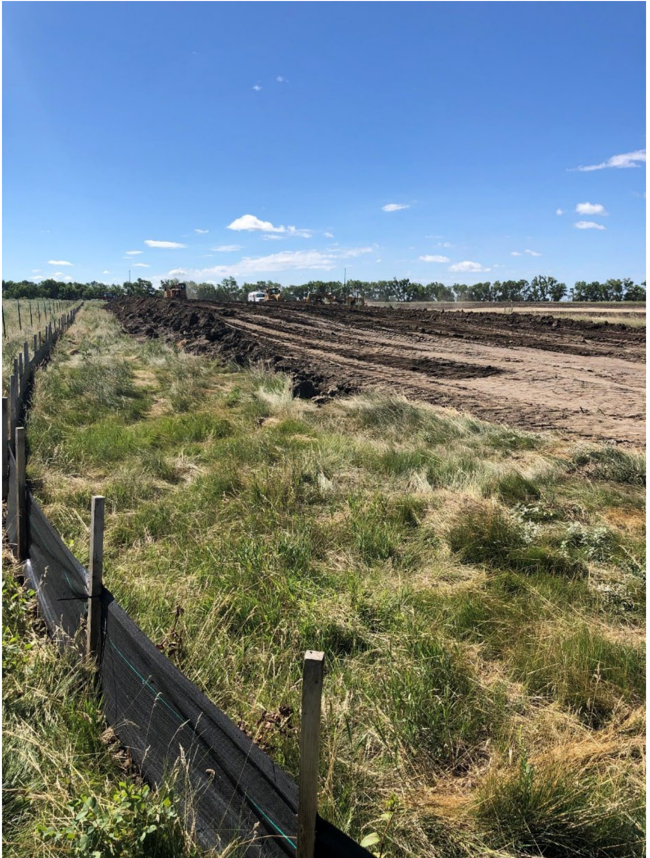
Figure 15: Topsoil stockpile and silt fence in the East Youngtown Tract.
